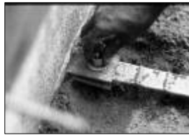
Reinforcing Strips are bolted to the facing panels
