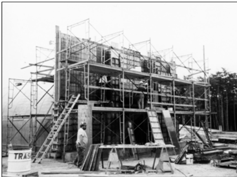
Built-in-place formwork slows construction of the end walls
