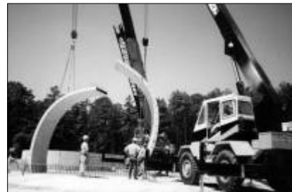
A standard 80-ft long magazine arch can be erected in one day
