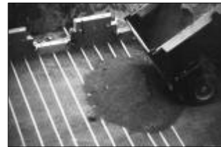
Backfill is spread and compacted
