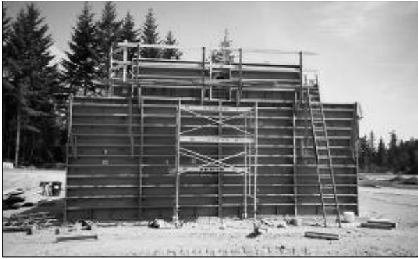
Modular formwork speeds construction of the portal walls
