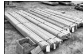
Soil reinforcements are shipped To the jobsite in bundles
