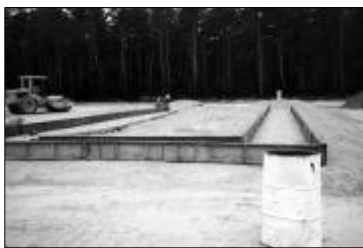
The arch footings are formed and poured in place
