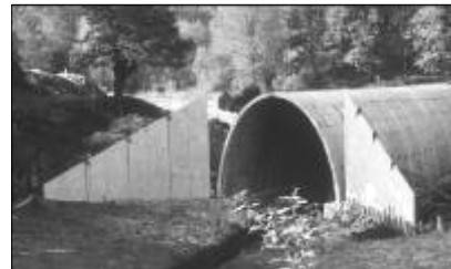
Full-height precast wing wall panels speed construction
