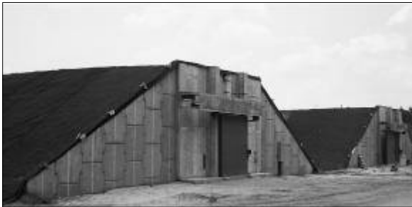
Erosion control blanket installed prior to final earth cover
