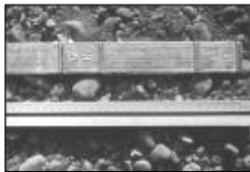
Soil Reinforcing Strips measure 50mm wide x 4mm thick
