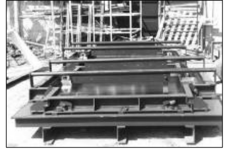
Reinforced Earth Wall precasting forms
