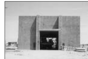
Completed Portal Wall
