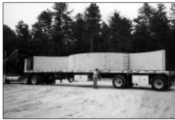
3 arch panels comprise a truckload, while 20 to 30 wing wall panels comprise a truckload
