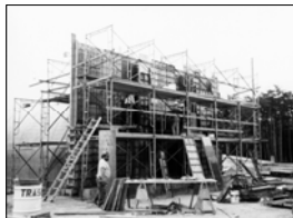
Built-in-place formwork
