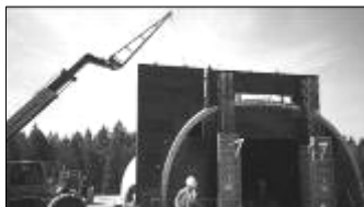
Prefabricated modular formwork
