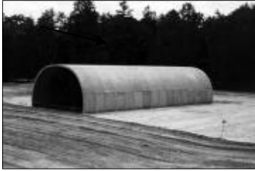
Completed TechSpan Arch
