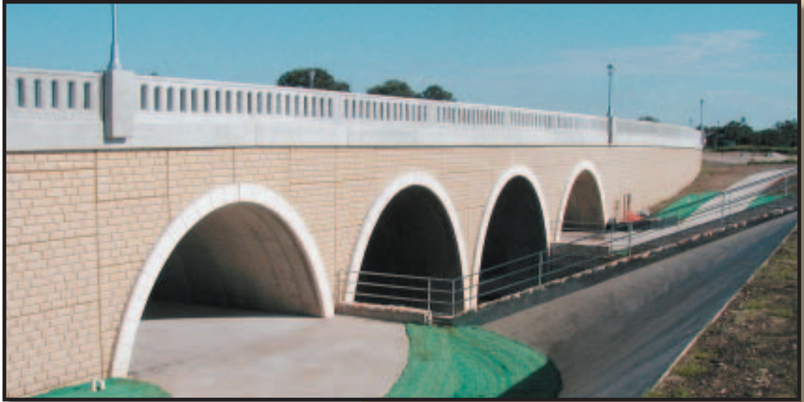
Discovery Blvd. Cedar Park, Tx. Chiseled Limestone Finish
