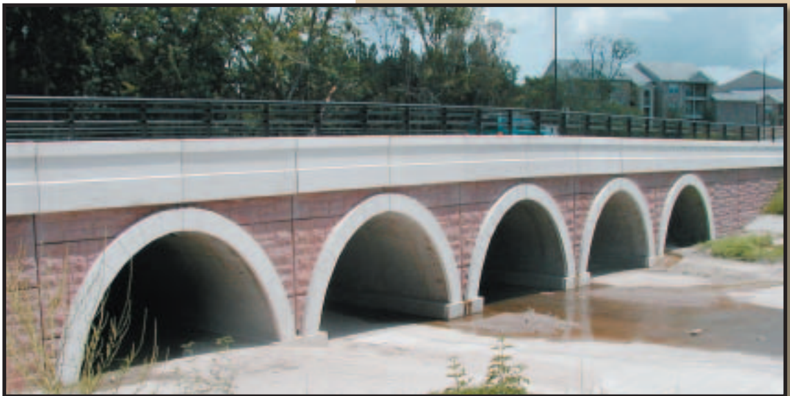
George Bush Drive East. College Station, Tx. Ashlar Stone Finish
