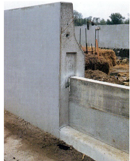
Piano Wall allows a smooth transition to other retaining walls on the same project
