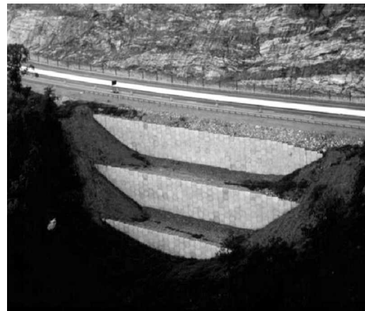
Figure 1b. Tiered Wall US 23 Unicoi County, Tennessee
