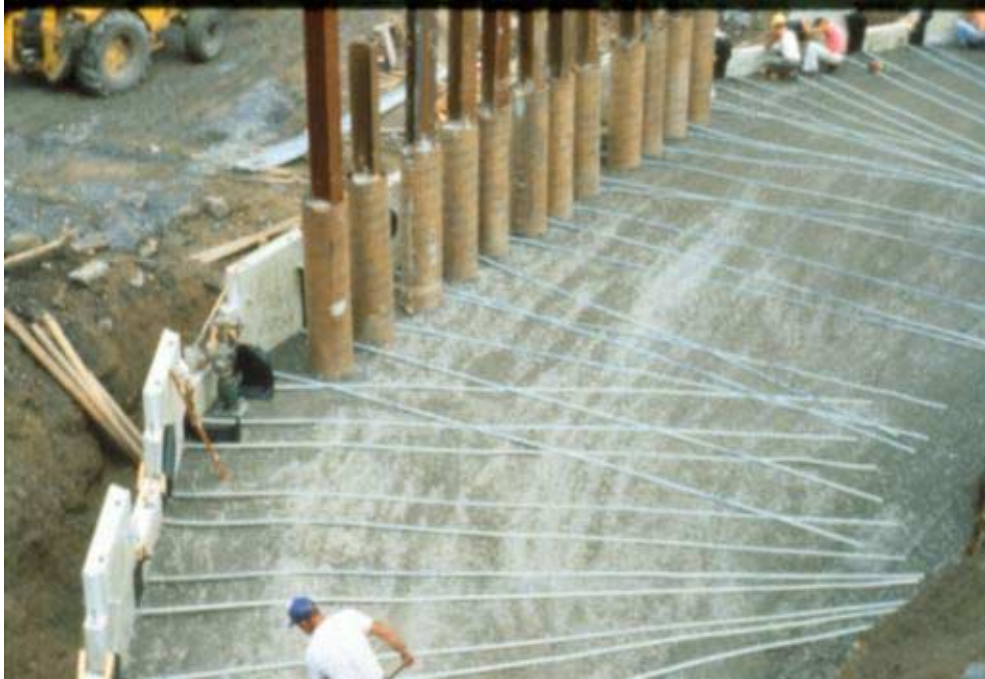
Pile Supported Abutment with reinforcing strips skewed around piles.
